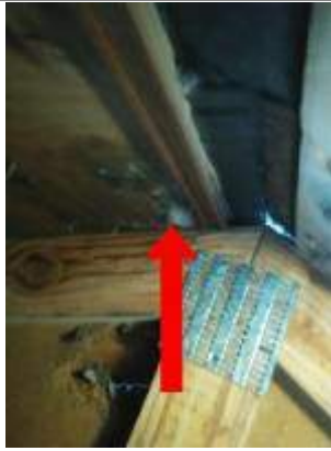
East at Ridge water entry point
