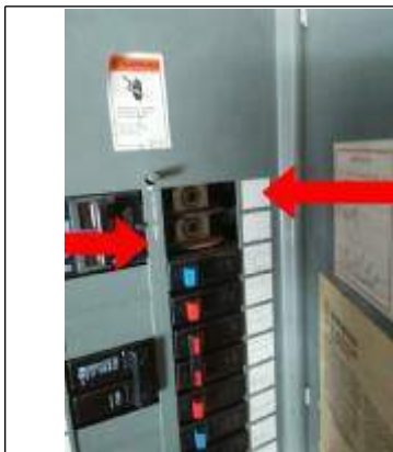
Missing knockouts
